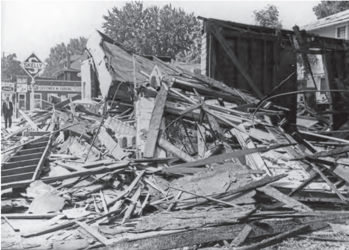
“In a second round of violence in August 1966, a fire set by an arsonist caused an explosion which leveled this café near Omaha’s racially disturbed Near North Side 8/3. An adjacent service station and nearby homes were damaged.” United Press photo, August 3, 1966. NSHS RG2467-24
